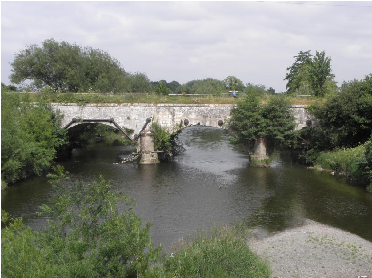
Vyrnwy Aqueduct Montgomery Canal – note the reinforcing ties
