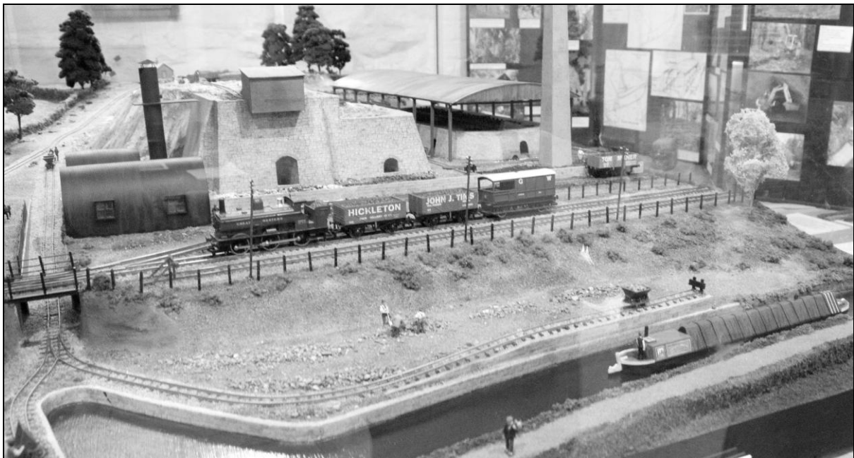
Model showing the relationship between the Hoffman Kiln, the Limeworks, the canal, railway and tramways
