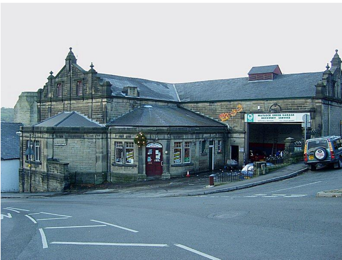
Matlock Steep Tramway - 'depot'
