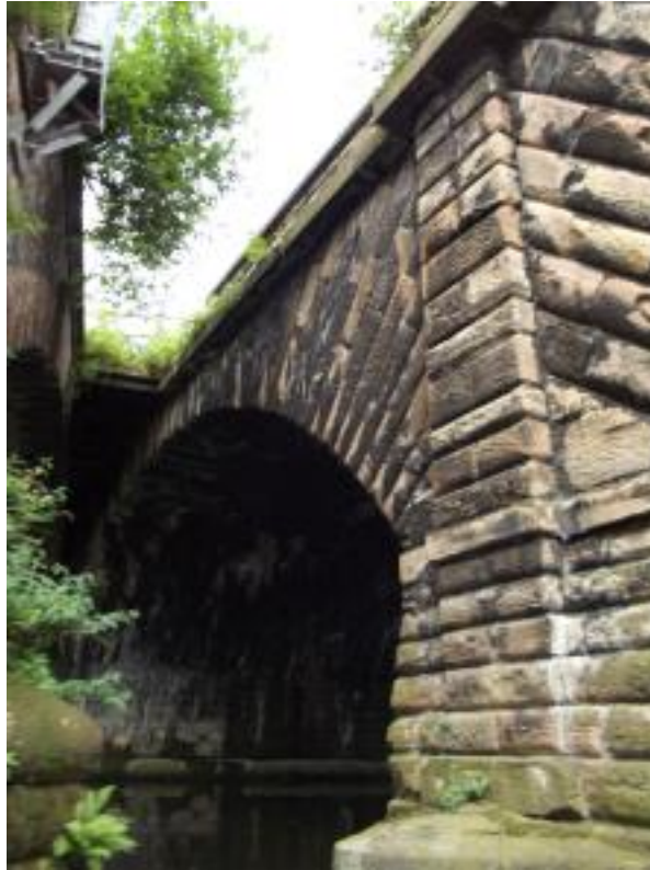
Stephenson's skewed River Irwell railway bridge of 1830 seen from the river.
